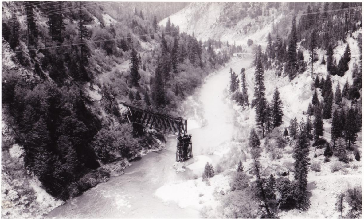
The tressel at Paxton after it's destruction; 1938.
