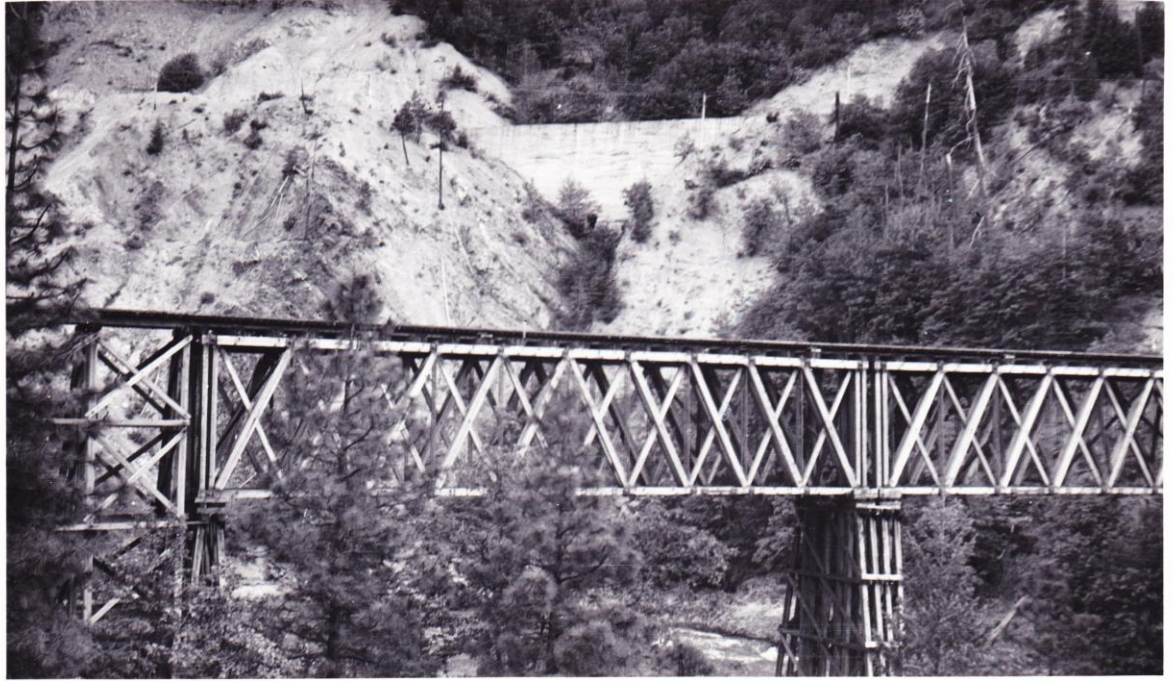
The tressel at Paxton as it appeared in May, 1938.
